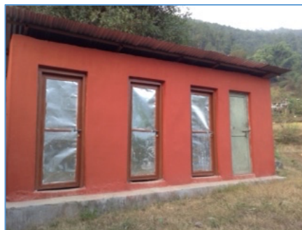
New toilet block
